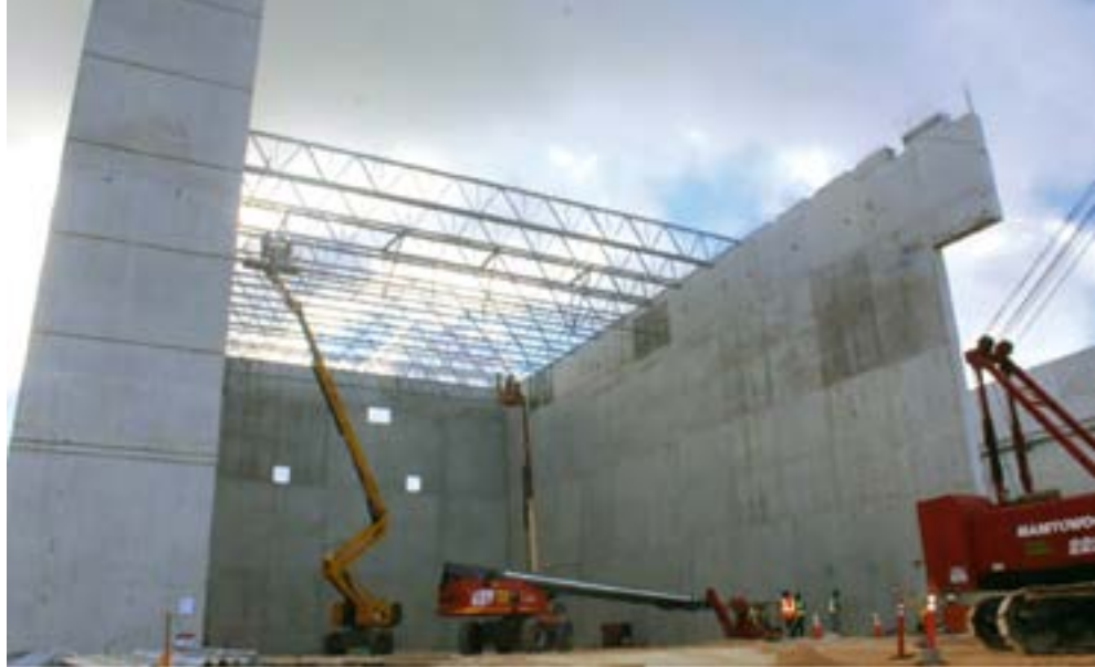
Black Construction Corp. is building the 260 Corrosion Control Hangar on Guam as part of the island's ongoing surge in military construction.
