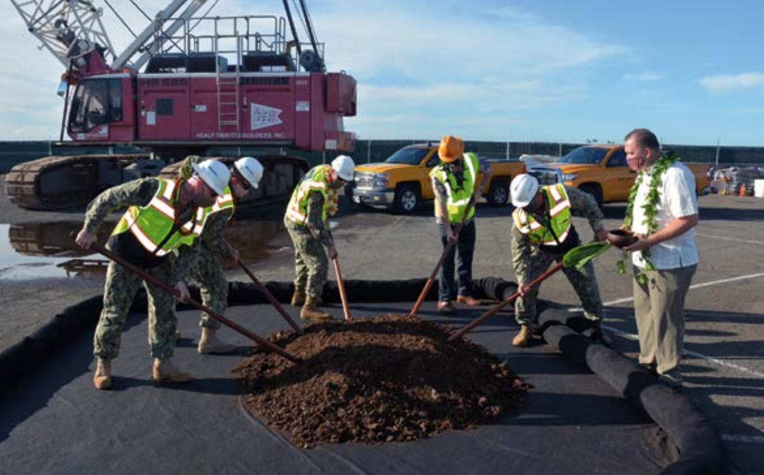
Groundbreaking and blessing at a recent NAVFAC Hawaii project
